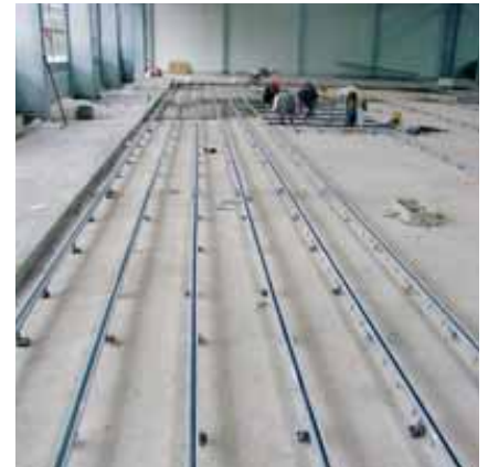
Anchor channel JTA W 74/48 for fixing machine elements. Absorption of dynamic loads through the W-profile and high loads possible.
