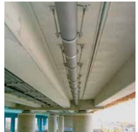
Pipe suspension under a bridge. Short anchor channel pieces for series fixings with optimum possible adjustment.
