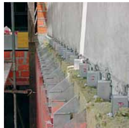
Installation of facade brackets on the anchor channel JTA K 38/17-200. Exact alignment along the anchor channel possible.
