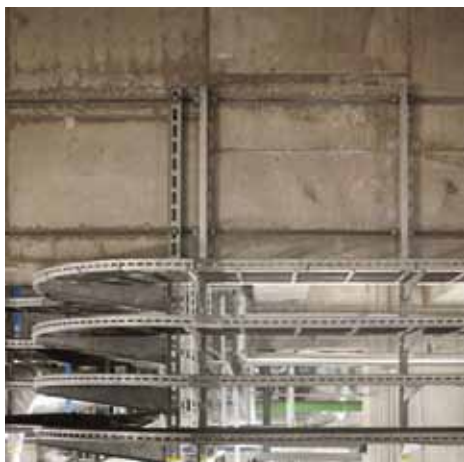
Attachment of Cable Support Systems
